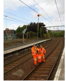
The 0480-6001 camera head has been designed and qualified to operate safely and seamlessly with live high voltage wires (29Kv AC as standard or higher if required) and connects to a client supplied fibre glass "Hot stick" pole (10m max) with optional angled knuckle adapter. Each camera is supplied with a removable robust adjustable-output LED lighting unit.
